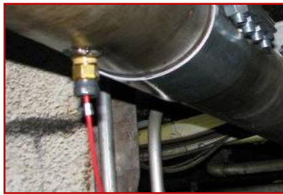
Fig 24: Threaded Sensor installation detail
