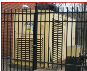
Fig 16: Standby Generator
