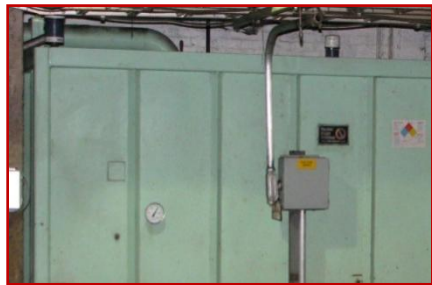
Fig 23: Dry End Reservoir
